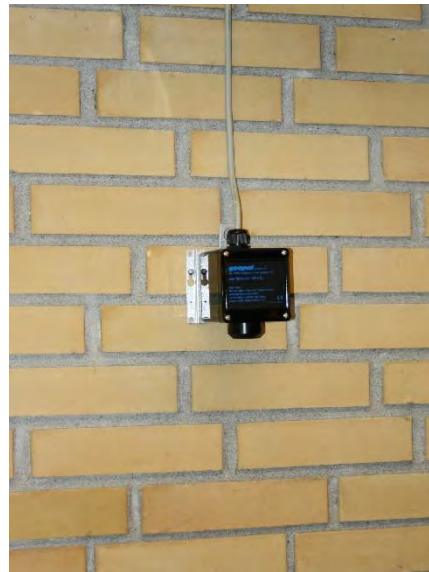
Figure 2 For flexible wall mounted installation, use wall bracket, part number: DET-1050.
